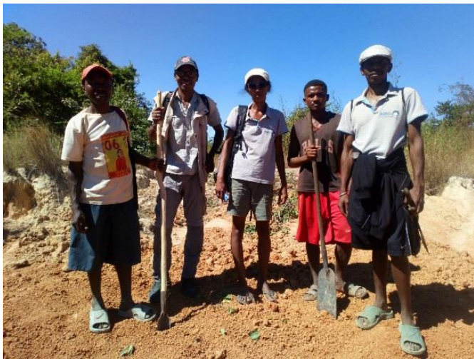
Photo 12 : AEEL team working on road levelling
